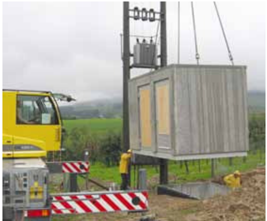
Montage Transformatorenstation Stiigere, Freienwil
